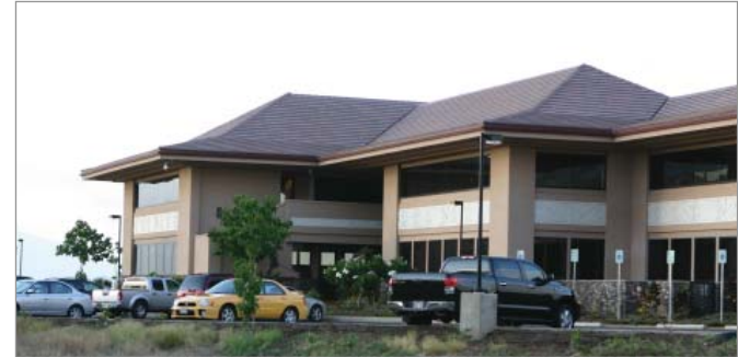
Park Plaza Building in MRTP
